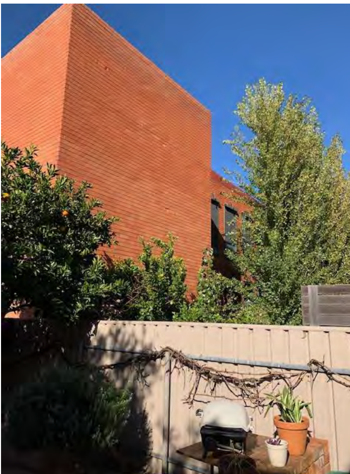
Photo 4 – View of rear wall of 3 storey office building at 17-21 Bagot Street
