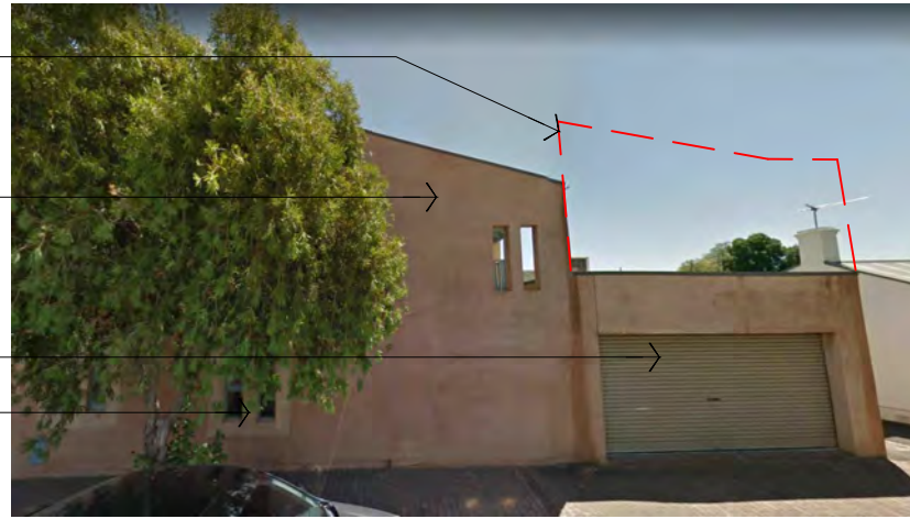
Tower St North - Existing
