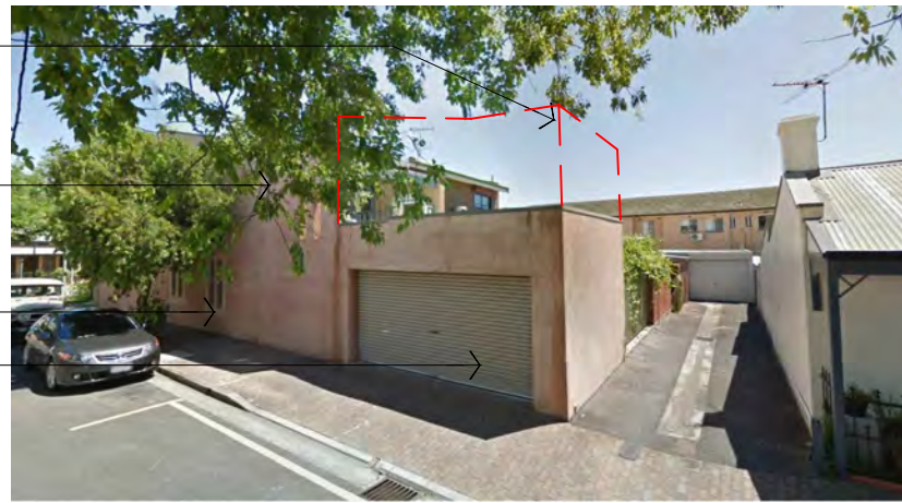
Tower St North - Existing
