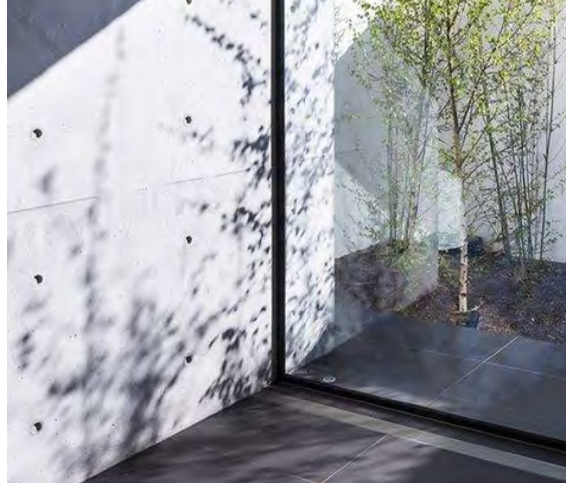
CE IN-SITU OFF FORM CONCRETE WALLS GL CLEAR GLASS / BLACK ALUMINIUM WINDOW FRAMES
