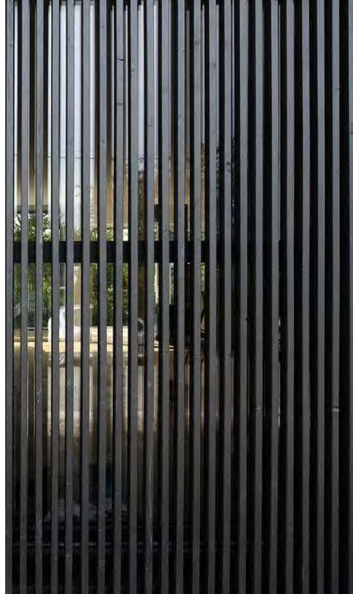
EXAMPLE OF SCREENING WITH GLASS BEHIND
